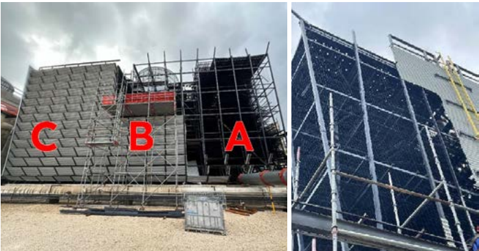
Figure 2: Cooling Tower Undergoing Diagonal Brace Fix (left), Diagonal Brace Fix Overview (right).
